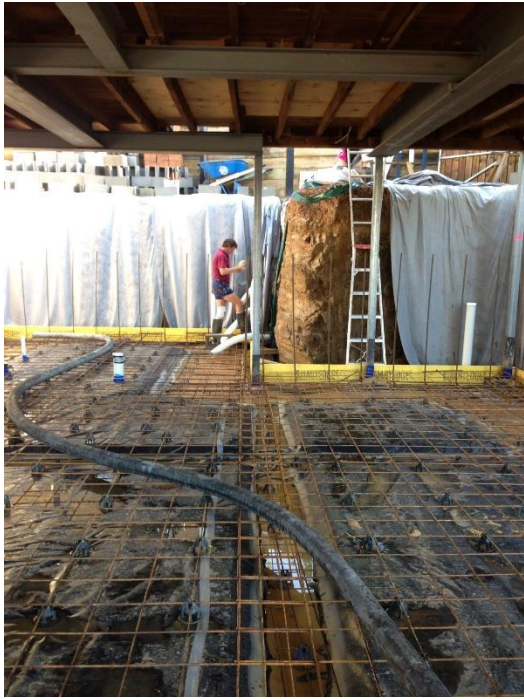
The slab ready for pouring. Note that the Capiphon has been covered with more coarse sand and plastic sheeting before the reinforcing has been laid.
